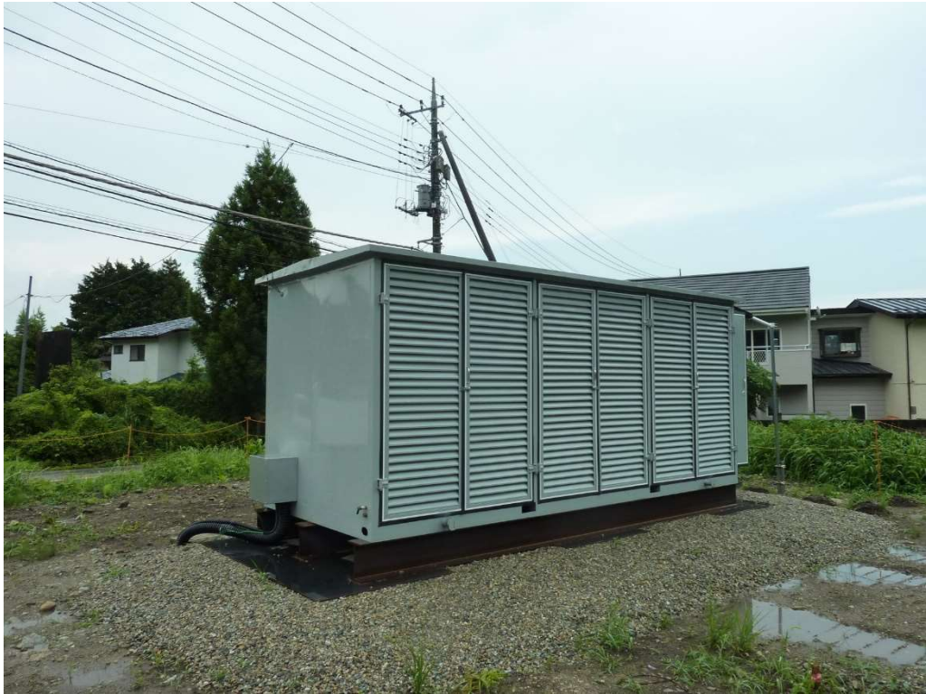
Containerized data center (exterior)
